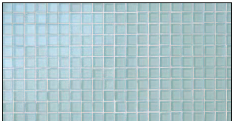
STEP 12 After 24 hrs, use a clean dry cloth or other cleaning solution to remove the excess grout haze.
